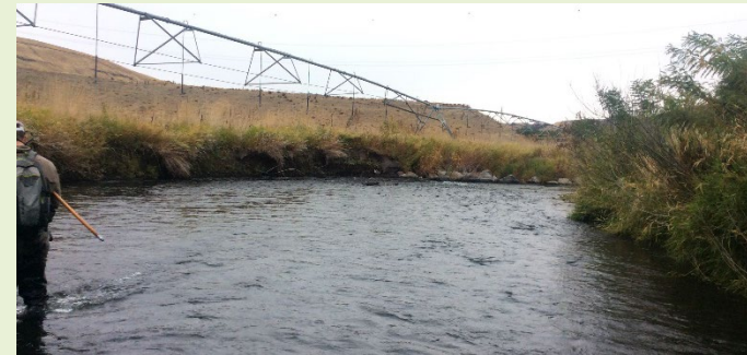
Project Area 44 PA 44 mid-reach, looking downstream at erosion into a field on the left bank on the outside of a meander bend.
