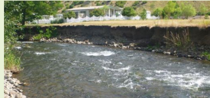
Project Area 16 Photograph taken from the 2011 prioritization showing bank erosion adjacent to a private infrastructure, looking across at the right bank.
